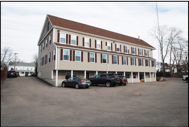
View of Rear
