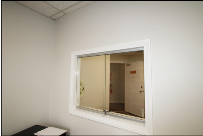
2nd Floor Office
